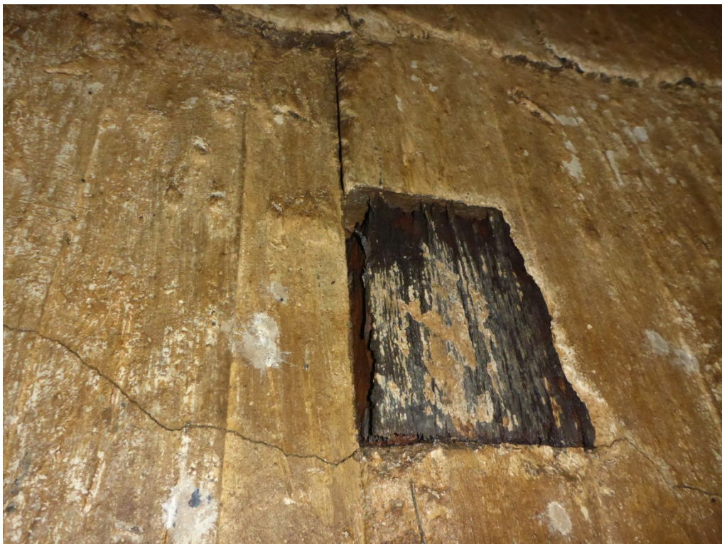
Figure 8: Existing Form Penetrations
