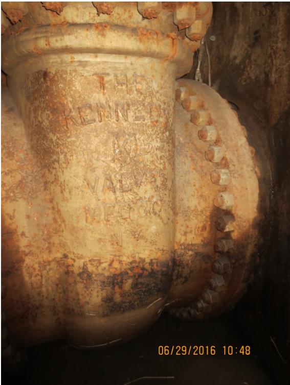
Figure 2 - Existing 1200 mm Gate Valve
