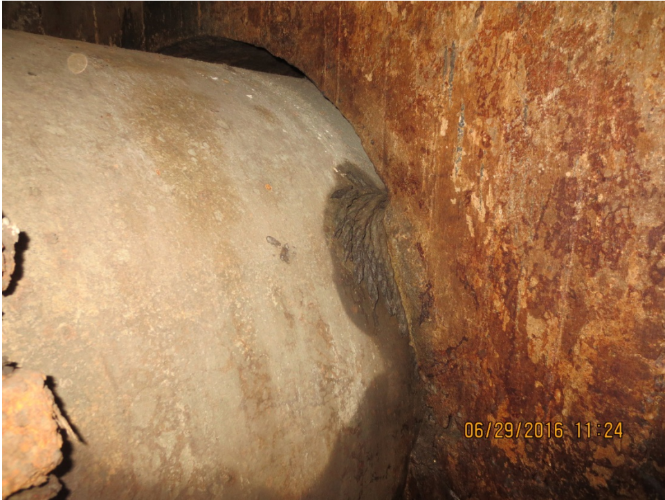
Figure 5: Existing Pipe Penetration
