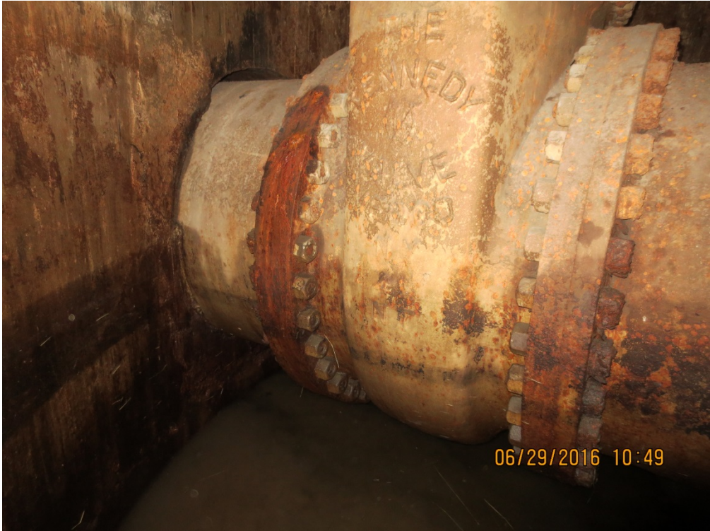
Figure 1 - Existing 1050 mm Gate Valve
