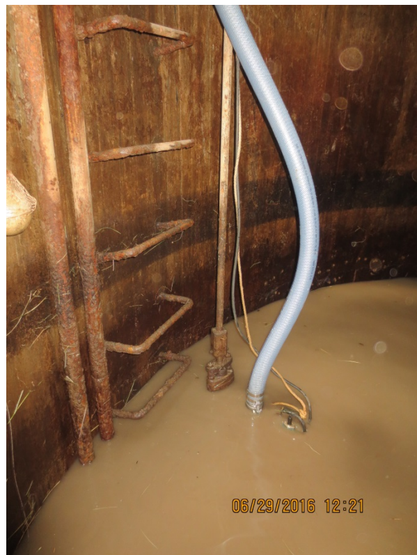
Figure 4 - Existing 150 mm Drain Valve
