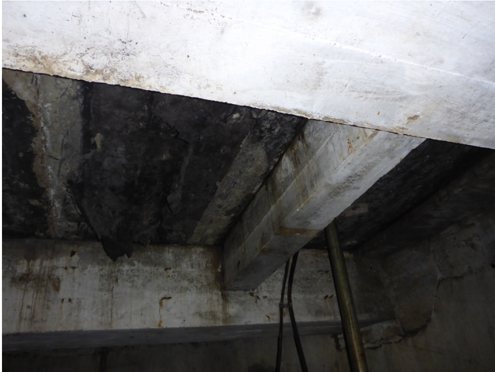
Figure 7: Existing Roof Structure
